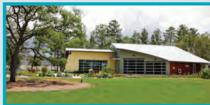
Movement Studio & Demonstration Kitchen
